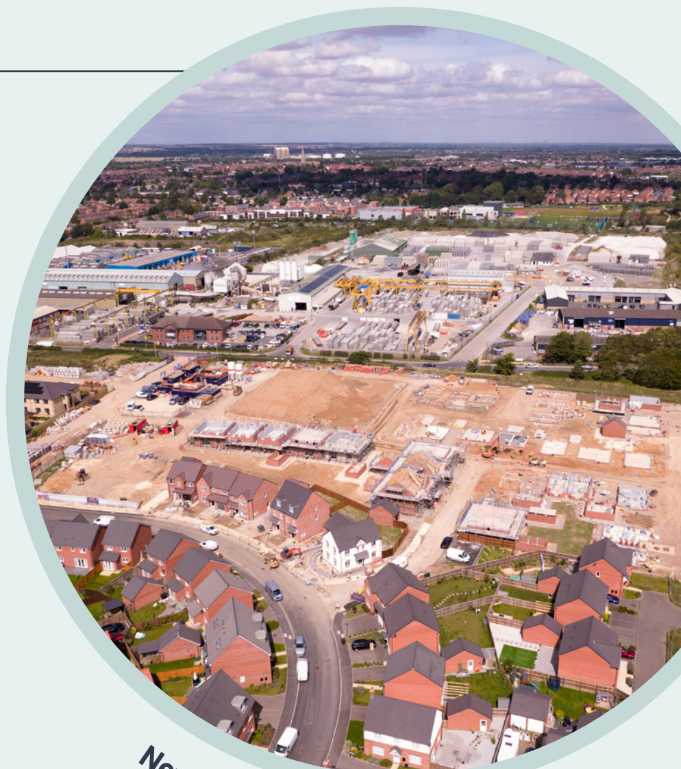
New homes under construction
